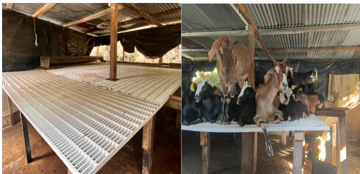
Raised FRP Slatted floor/Platform for Goat shelter
