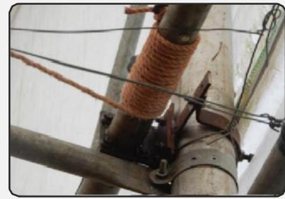
**Clamps and nut bolt fitting system to the rotating GI pipe fitting**
