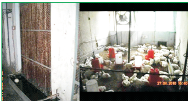
Fig. 18 .Fan-Pad cooling system
