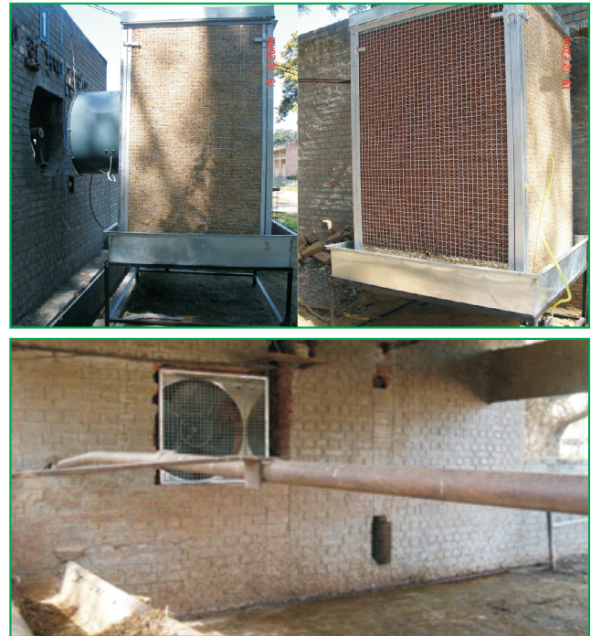
Fig. 25 .Fan-pad system fitted in the GADVASU shelter
